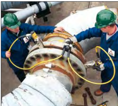
◀ Two FSH-14 spreaders used simultaneously with Enerpac handpump, hoses and AM-21 control manifold.
